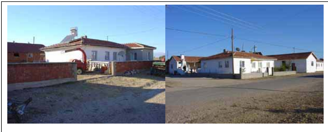
Post-disaster houses in Gencali Village with additional parts
